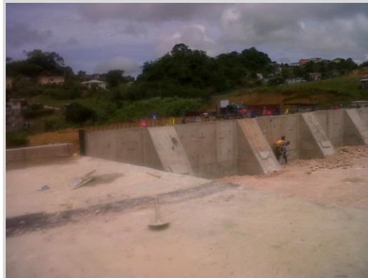
Picture 1 A section of the Christiana Development Road Project
